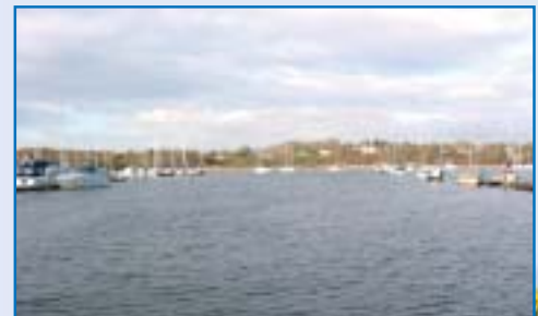
Relocation of existing moorings
