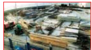
Building the Spinnaker Tower
